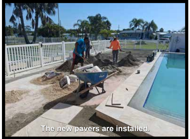
The work started with the new coping.
