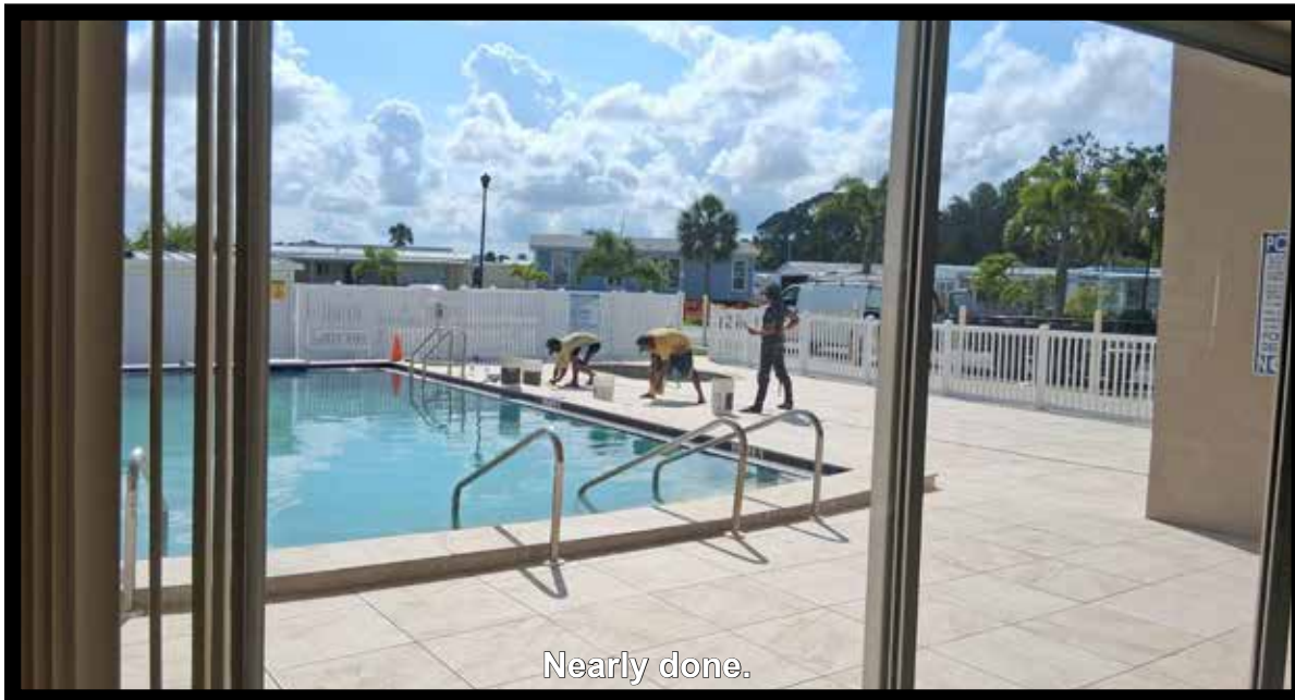
The work started with the new coping.
