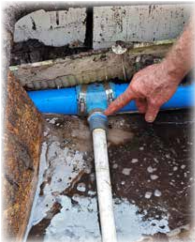
Repair to Water Line
