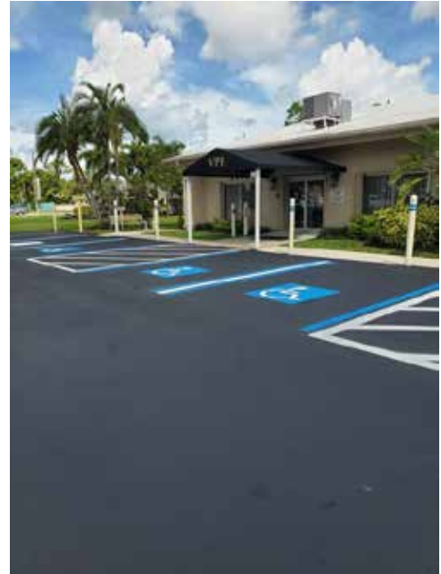
The roads have been sealed and repainted this summer
